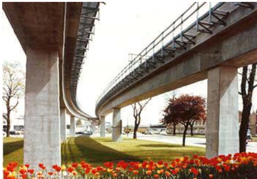
Clean lines and pleasing landscaping did much to make the project acceptable
