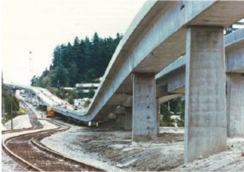
A depression in the freeform track alignment to make it less intrusive and avoid obstructing the scenic mountain views from a local residential estate
